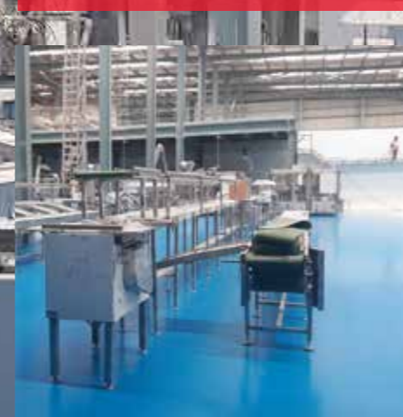
Allied Breweries Hyderabad, India Bottling & Packing Halls Nitoflor SL3000 UT in RAL5012 6,200m 2 , May 2017
