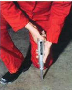
Schmidt hammer test
