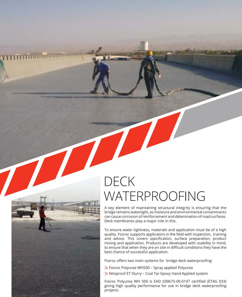
The rapid spray application provides high productivity especially beneficial for large bridges where construction times can be kept to a minimum. Polyurea technology provides excellent waterproofing, crack bridging, elongation, puncture and chemical resistance found in typical bridge structures. Hot rolled asphalt is laid on top of the membrane as the finished wearing surface.
