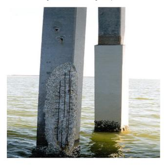
The Galvashield LJ system is a two piece 'Tongue and Groove' interlocking jacket assembly. It is positioned and held in place with non conductive fasteners and sealed moisture tight with an approved adhesive.
